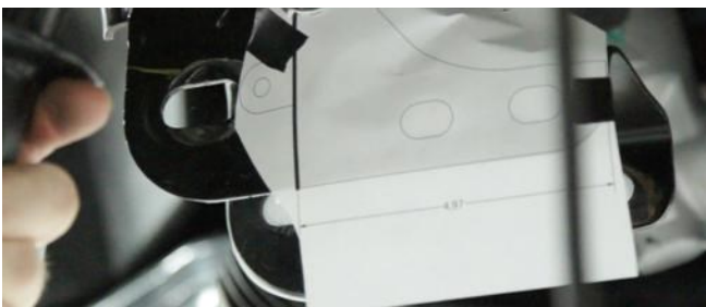
INSTALL THE TEMPLATES AND CUT
