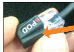
Be sure to keep protective cap on. Form a hook on the end of the fish line & wrap the connector with a little electrical tape
